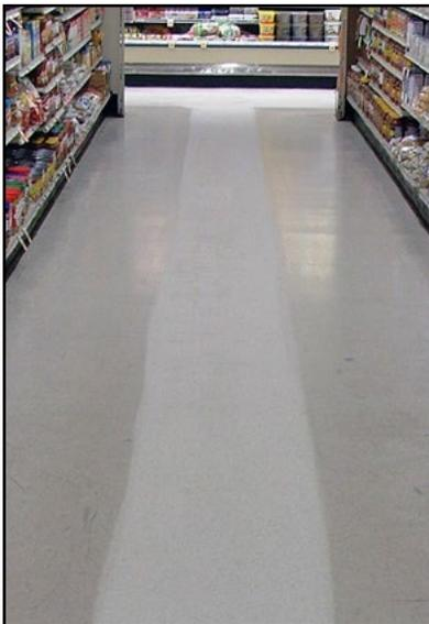
One pass with an orbital scrubber equipped with a surface prep pad
