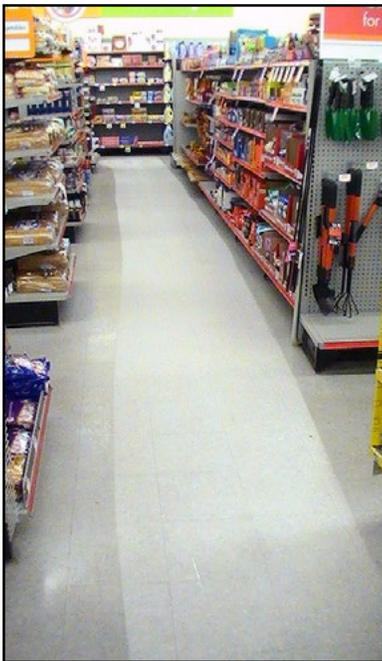
Finish removed with a 20-inch orbital scrubber using a surface prep pad
